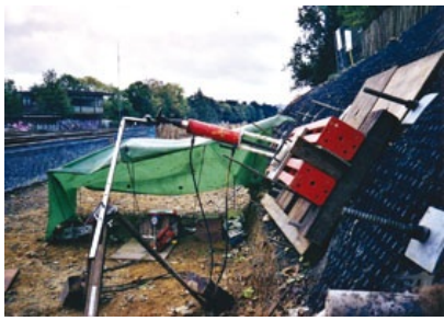
Testing of DYWI® Drill Hollow Bars for slope stabilization
