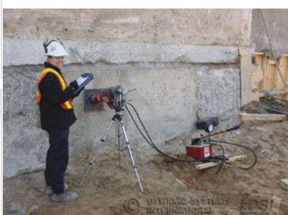
DYWI® Drill Anchor testing
