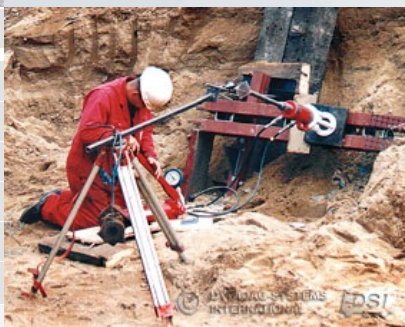
Testing of DYWIDAG Soil Nail
