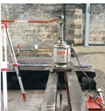
Tensile test on a temporary anchor pile
