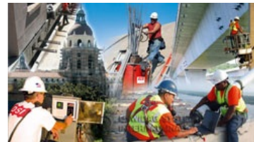
Structural Repair Solutions
