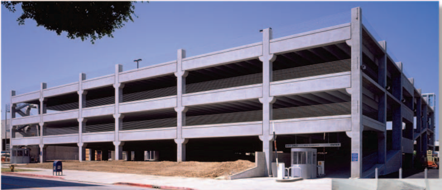
Wiltern Parking Structure, Los Angeles, CA
